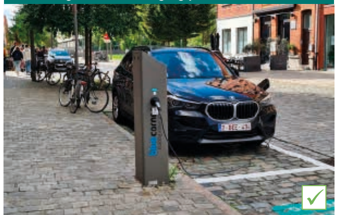
EV charging points should be designed into the public realm and not be added as an afterthought
