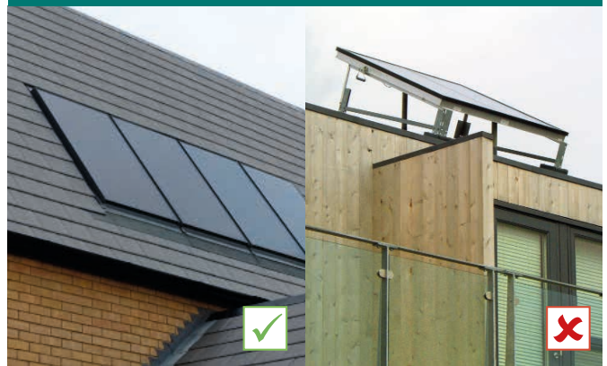
Photovoltaic panels should be well-integrated into the composition of the roof and ideally recessed. Additional installation frames will not be permitted.
