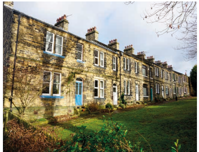
Good quality housing for mill workers, Akroydon
