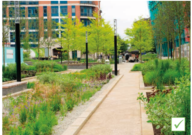
Green verge with biodiverse planting and rainwater attenuation - Sovereign Square, Leeds (Slow the Flow)
