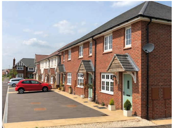
Frontages dominated by car parking, with little or no landscaping
