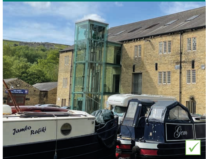
Use of contemporary materials integrating sensitively with an historic building
