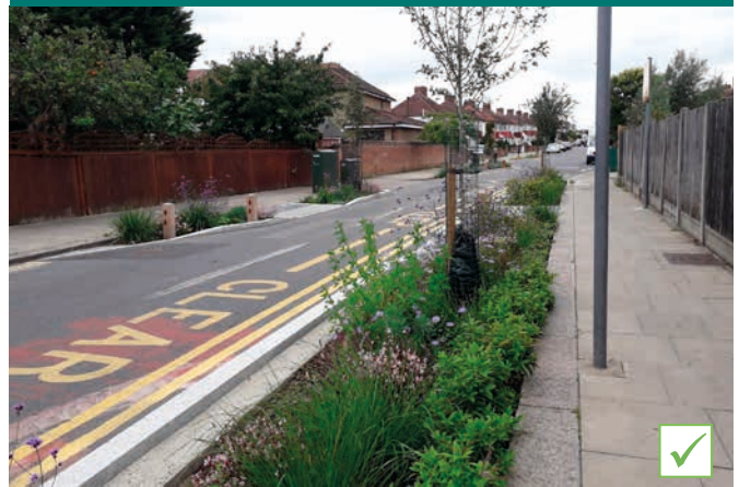
Green verge with biodiverse planting and rainwater attenuation lines the street
