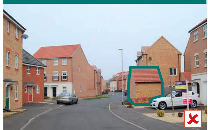
Location of substation
