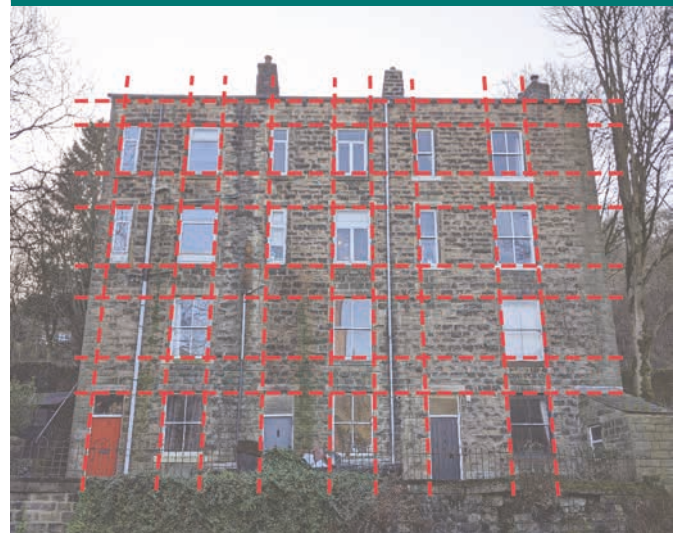
Regular arrangement of windows and doors
