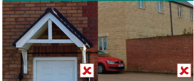
Poor quality GRP porch with inlegant detailing.
