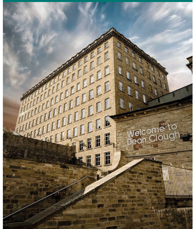
Conversion of Victorian mill buildings
