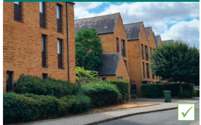
Landscape treatment of substation
