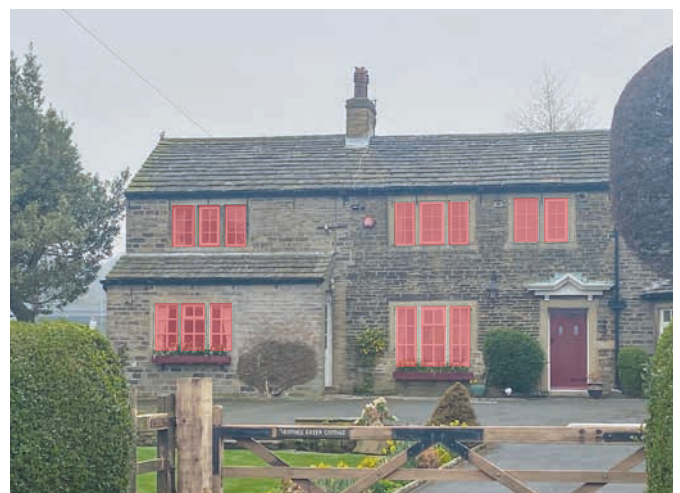
... or in rural areas, arranged in bands of smaller vertically proportioned windows, separated with stone mullions
