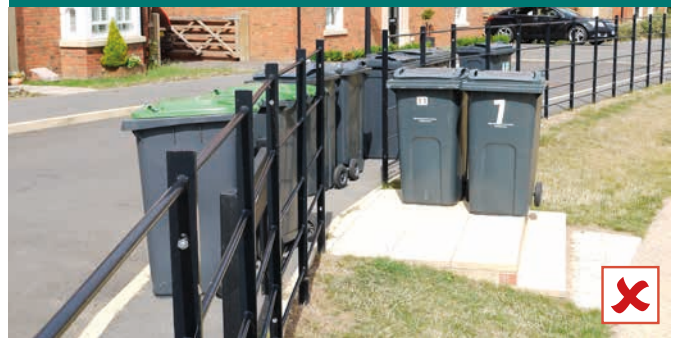
Lack of provision for bin collection
