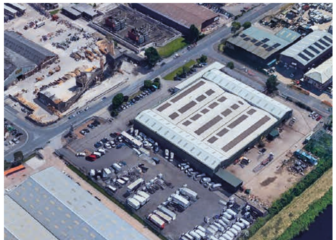
Industrial/Commercial Area, Brighouse
