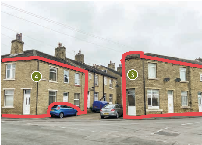
Building corners and ends that visually bookend terraces, and generously engage with and overlook the street.
