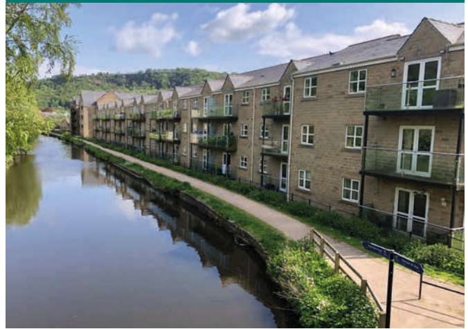
Active frontage along the canal
