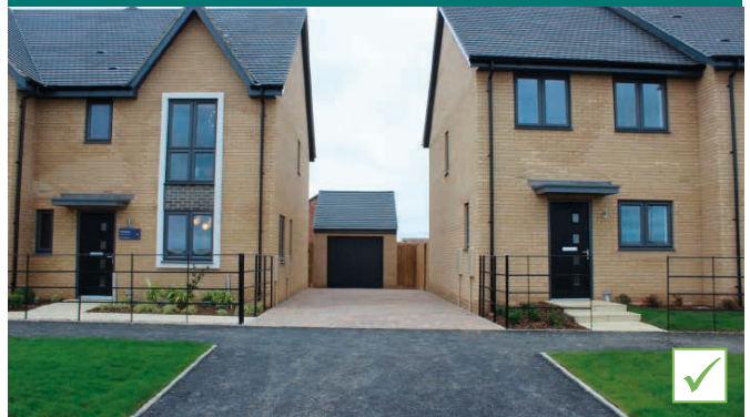
Well integrated garage to ensure parked vehicles sit behind the building line
