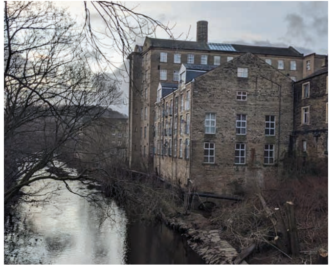
Old Cawsey, Sowerby Bridge
