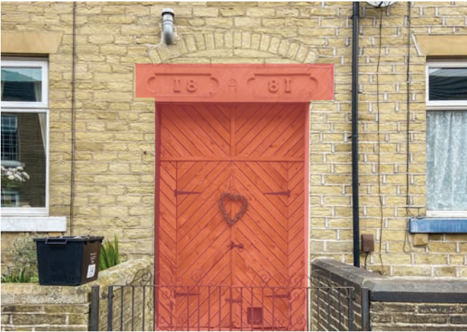
Generous passageways in runs of terraced to allow access to rear gardens
