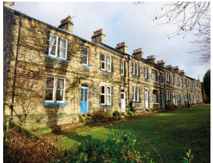
Good quality housing for mill workers, Akroydon
