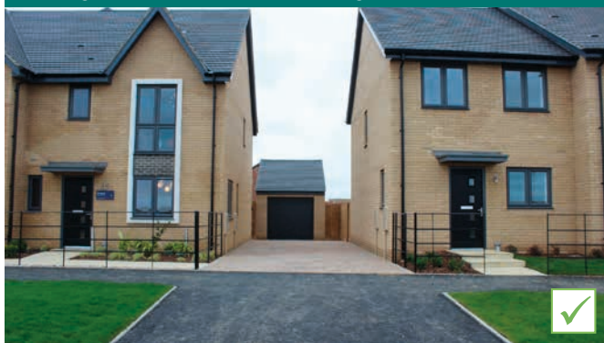
Well integrated garage to ensure parked vehicles sit behind the building line
