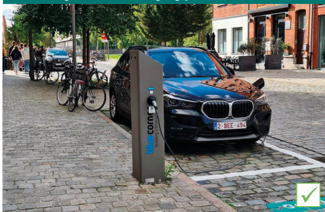
EV charging points should be designed into the public realm and not be added as an afterthought
