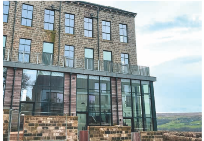
Materials that are complementary to local stone such as natural timber are sometimes used on modern buildings
