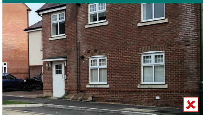
Lack of defensible space will not be acceptable
