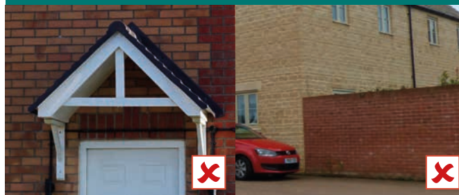
Poor quality GRP porch with inelegant detailing.
