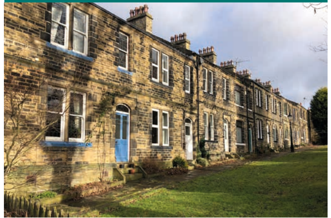
Identify the key characteristics of the surrounding landscape and buildings to inspire design proposals
