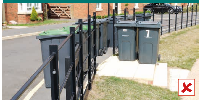
Lack of provision for bin collection
