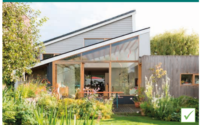
The new extension follows the pitch and geometry of the existing building (Gagarin Studio)
