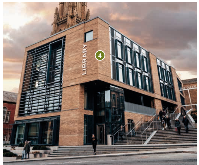
Contemporary architectural approach using carefully considered materials which are different but complementary to surrounding historic architecture.
