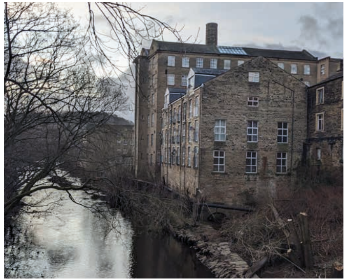
Old Cawsey, Sowerby Bridge
