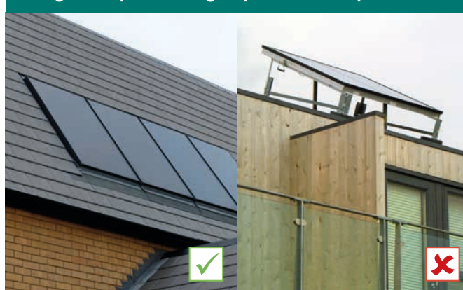
Photovoltaic panels should be well-integrated into the composition of the roof and ideally recessed. Additional installation frames will not be permitted.
