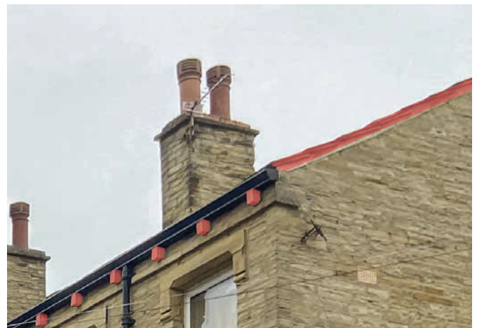
A consistent roof design with wet verge and stone dentils supporting the gutter
