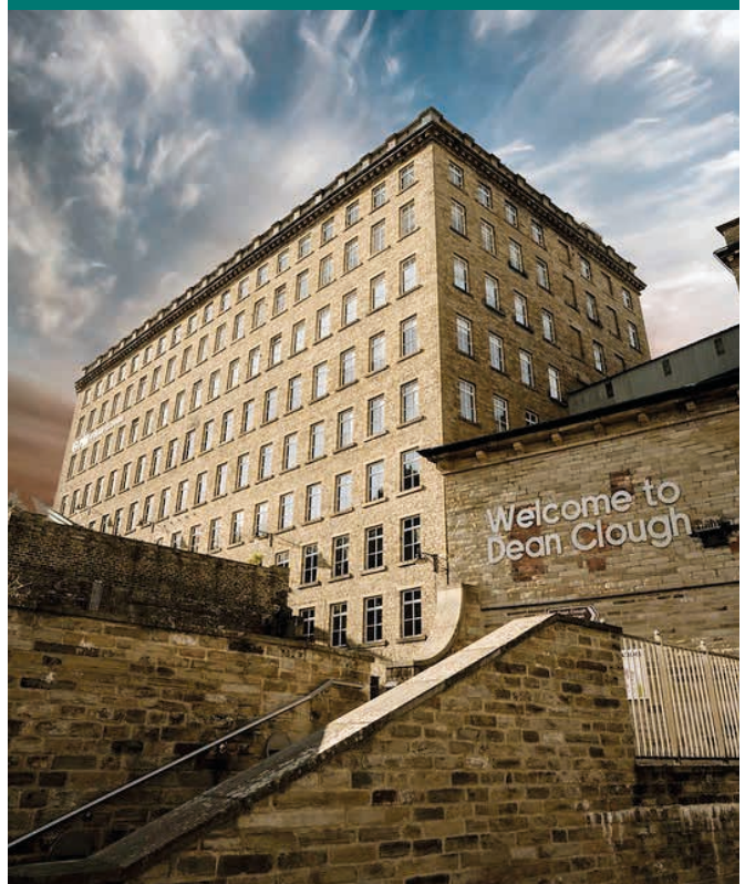
Conversion of 16 Grade II listed Victorian mills into a vibrant community of office, leisure and retail spaces - Dean Clough, Halifax
