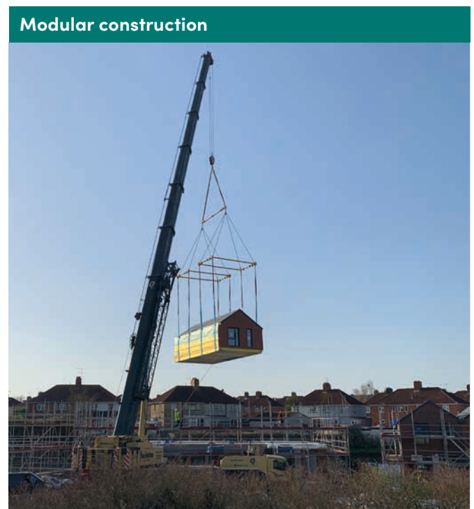
Housing modules manufactured off-site and quickly assembled on-site – Airport Road, Bristol.
