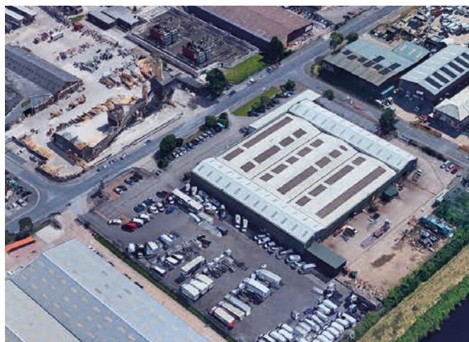
Industrial/Commercial Area, Brighouse
