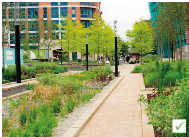
Green verge with biodiverse planting and rainwater attenuation - Sovereign Square, Leeds (Slow the Flow Ltd)
