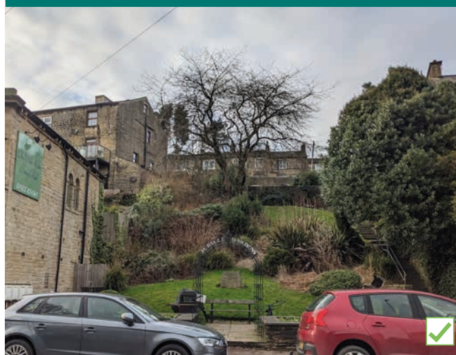
Attractive, incidental green space provided on steeply sloping site - Jubilee Gardens, Ripponden.
