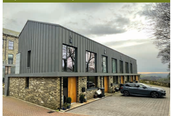
Adjacent new development to Old Town Mill
