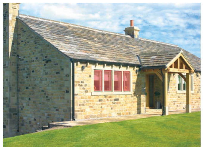
... or in rural areas, arranged in bands of smaller vertically proportioned windows, separated with stone mullions. (ADP Architecture and Design and Iain Richardson)
