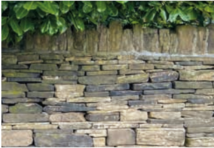
Local sandstone used for building and boundary walls, laid in a variety of bonds, with distinct variations in texture, shape and finish
